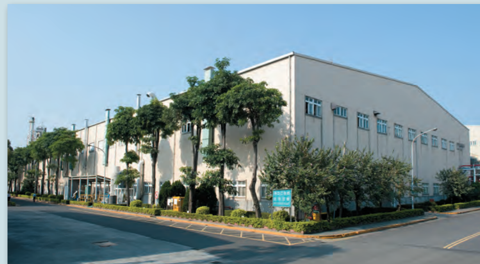
新港廠 Shin Kang switchgear plant
